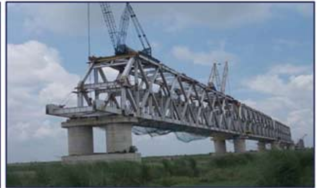
Assembly, erection / launching of triangulated steel girders for new rail -cum-road bridge across river Ganga at Patna
