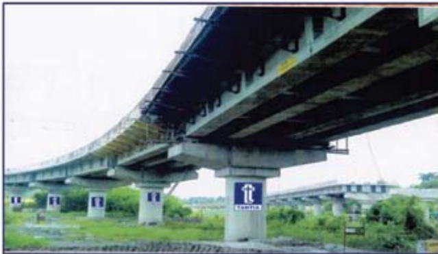
Execution of Civil Engineering Works of PSC via duct between Noapara and Dum Dum
