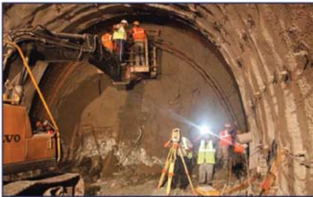
1.80 Kms long tunnel between Udhampur - Katra
